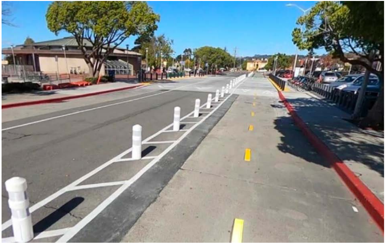
Separated bikeway at North Berkeley BART.
