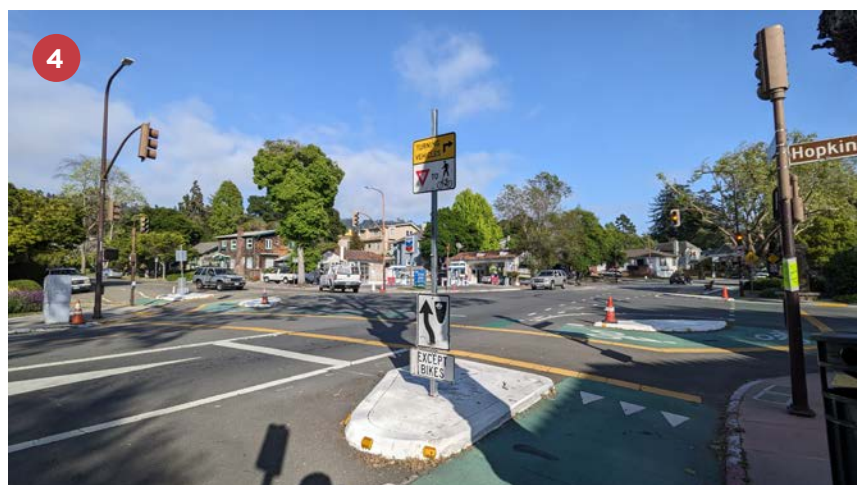
PROTECTED INTERSECTION on Hopkins Street at The Alameda (credit: Melanie Curry).
