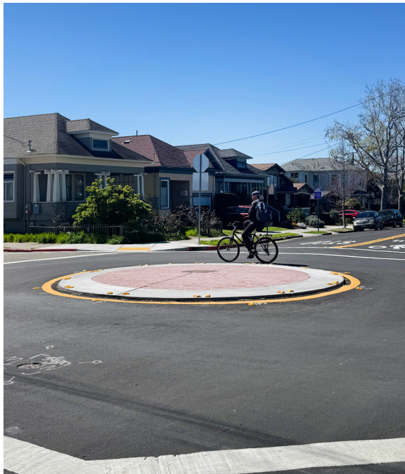
Fully Mountable Traffic Circle at Virginia Street and McGee Street (Source: City of Berkeley)
