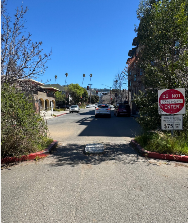
Newer Installation at Berkeley Way and Trader Joe's (Source: City of Berkeley)
