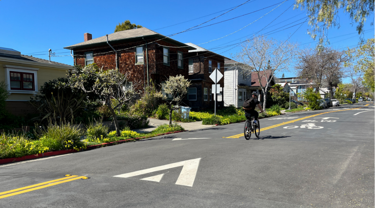
Speed Table at Milvia Bicycle Boulevard (Source: City of Berkeley)
