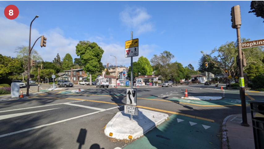
PROTECTED INTERSECTION on Hopkins Street at The Alameda
