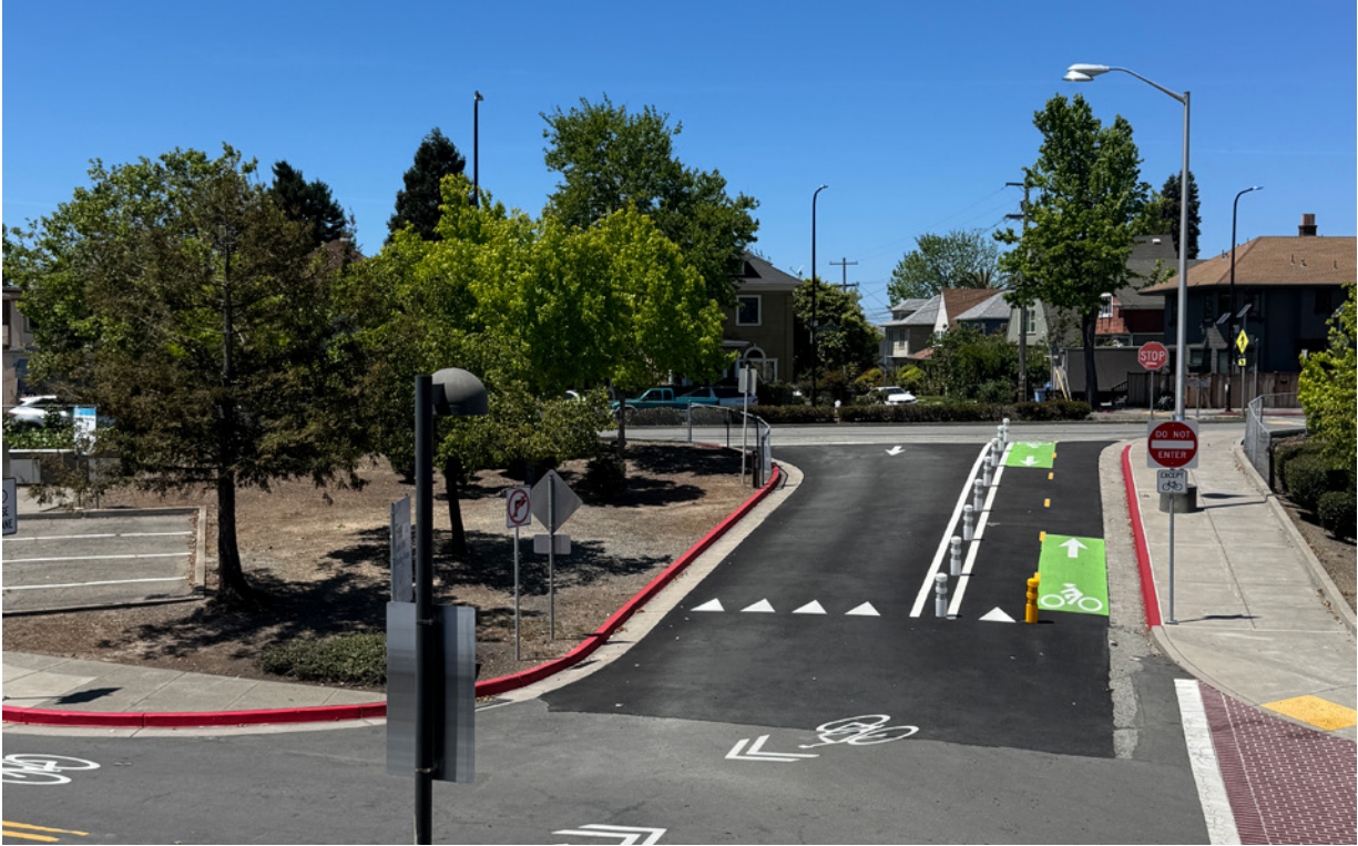
Two-way separated bikeway in the Ashby BART parking lot.
